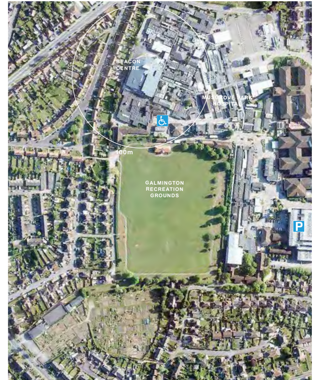
Site in the Context of Galmington Playing Fields and Musgrove Park Hospital
